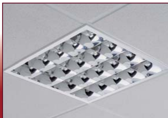
Example of converted emergency light
